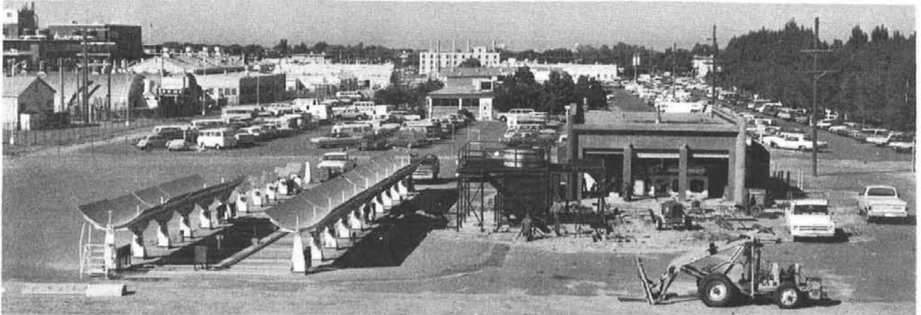
Figure 3-1. Solar Total Energy Test Facility (collector field lower left)
