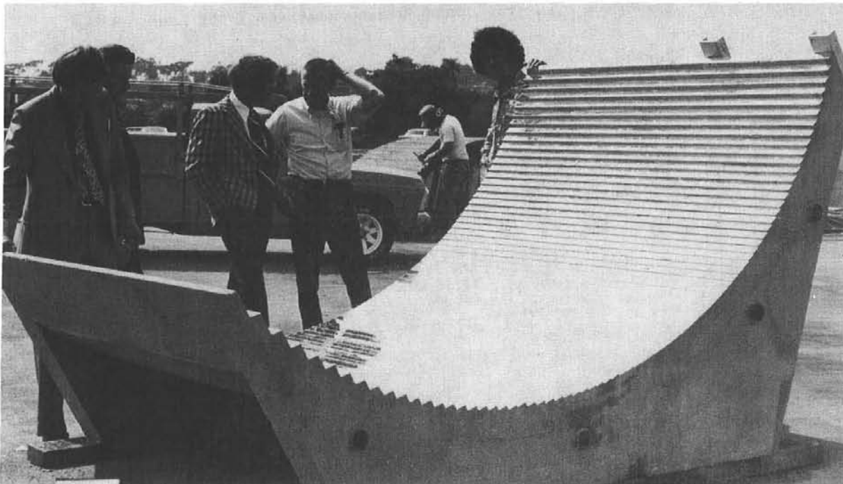
Figure 4-1. General Atomic Fixed Mirror Reflector
