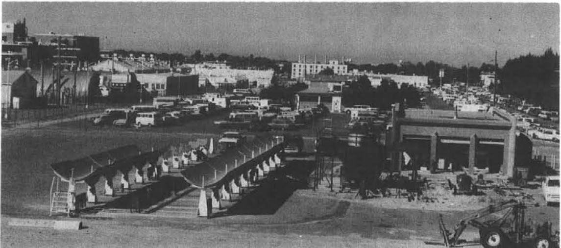
Figure 3-7. Present Solar Total Energy System Test Facility (collector field lower left)
