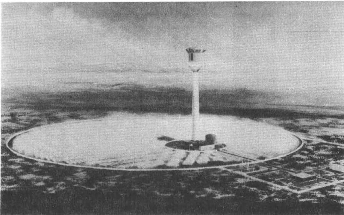
Figure 9. 10-MW e Solar Pilot Plant
