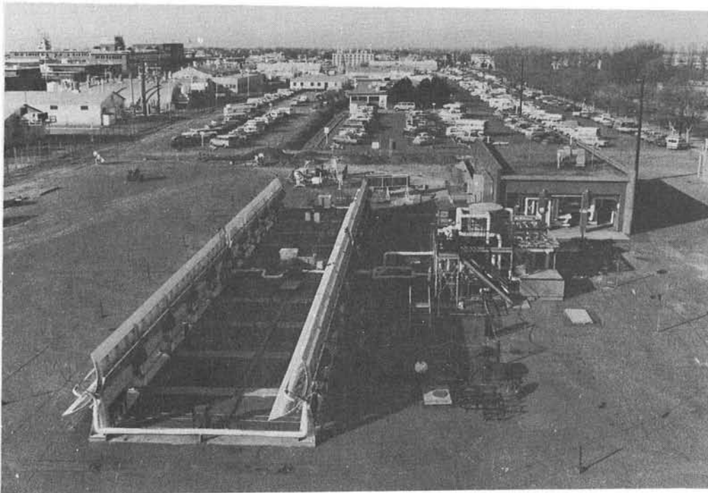
Figure 3. Solar Total Energy System Test Facility (STESTF) - January 1977
