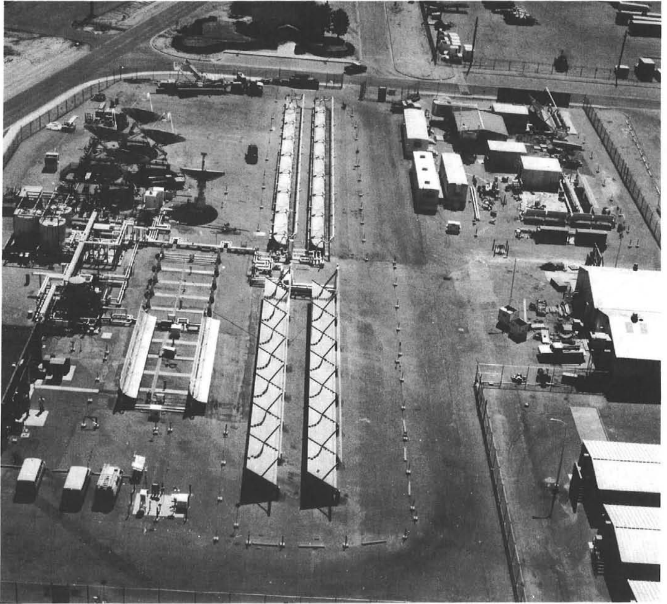
Figure 1(b). Aerial View of the MSSTF Taken from the West on 21 June 1979
