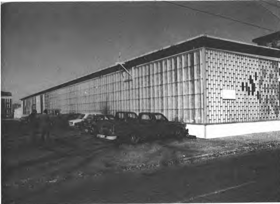
Figure 14-1. Direct-Gain Solar Heated Warehouse
