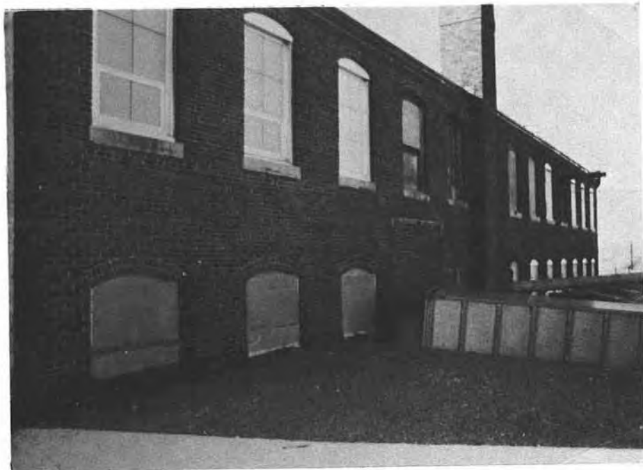
Figure 13-3. North Wall of Warehouse Showing Original Construction
