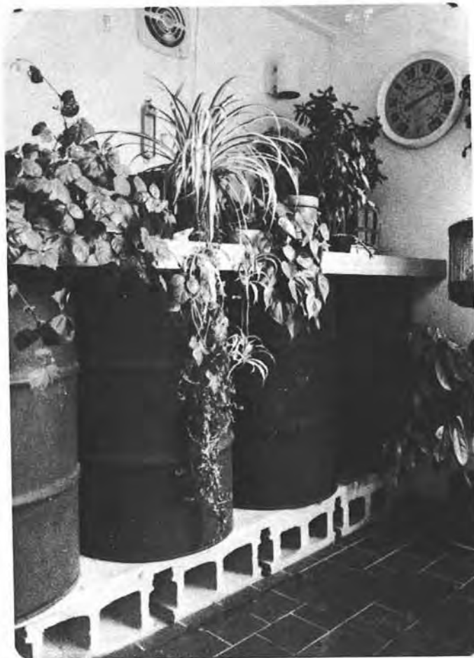
Figure 11-3. Water Drum Thermal Storage for the Hinesberg Greenhouse
