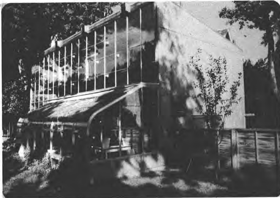
Figure 15-1. The Kelbaugh House
