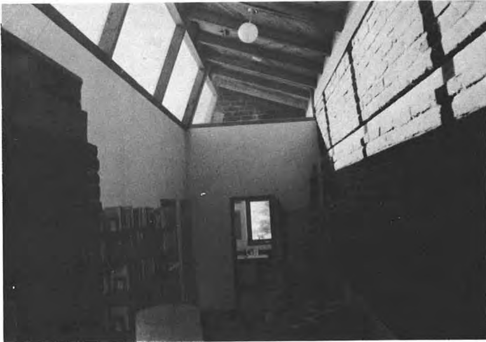
Figure 4-2. Sunlight from Clearstory Windows Falling on Adobe North Wall of the Williamson House
