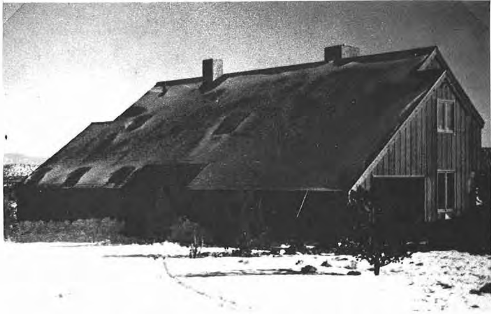
Figure 6-2. The North Side of the Shankland House
