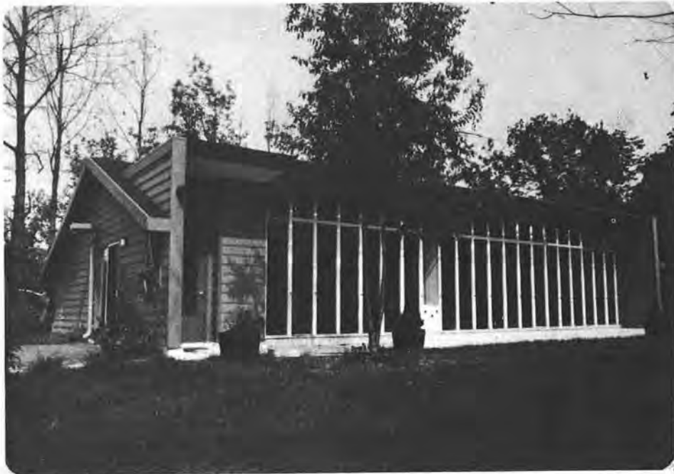
Figure 12-1. Exterior of Star Tannery House
