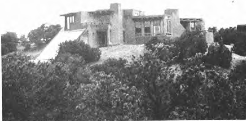
Figure 3-1. Exterior View of the Mark Jones House
