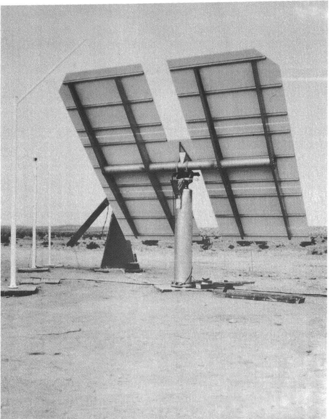
Figure 3. Prototype heliostat. (2)
