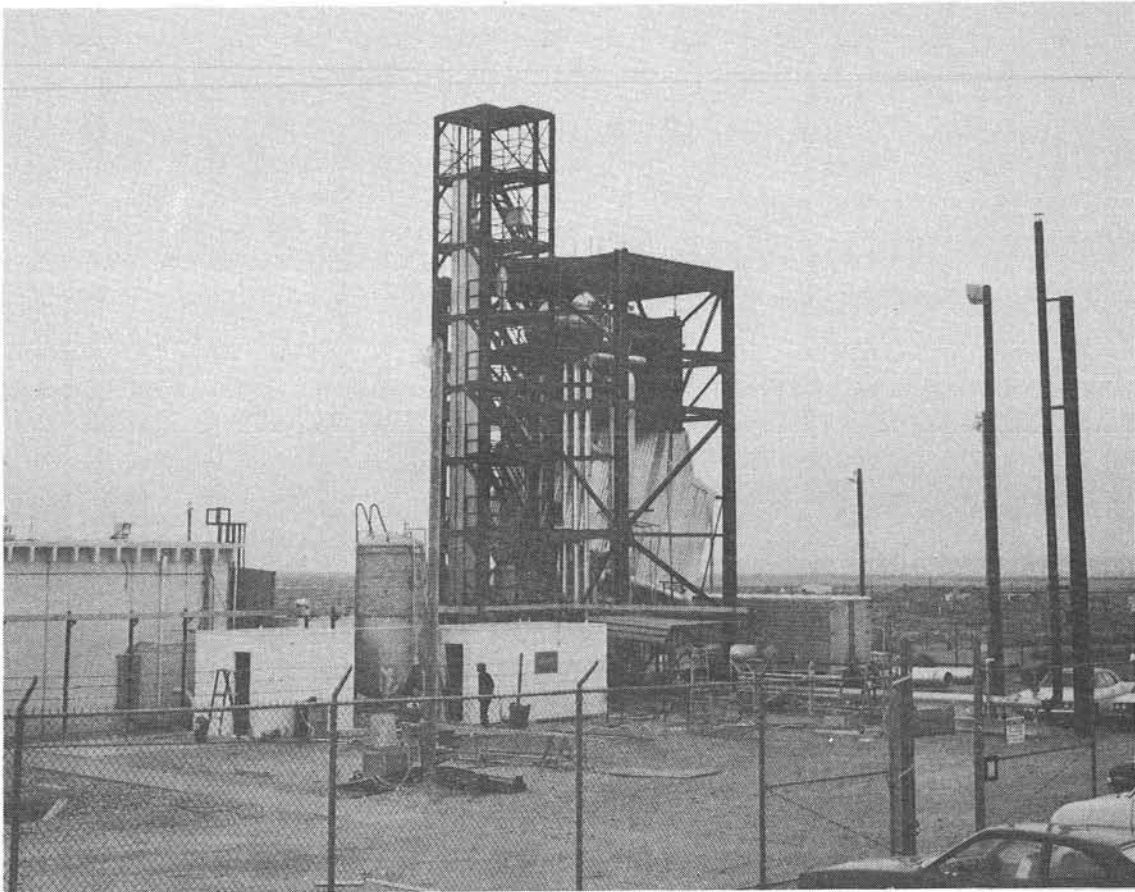
Figure 5. Five-Tube Water/Steam Receiver Panel Radiant Test
