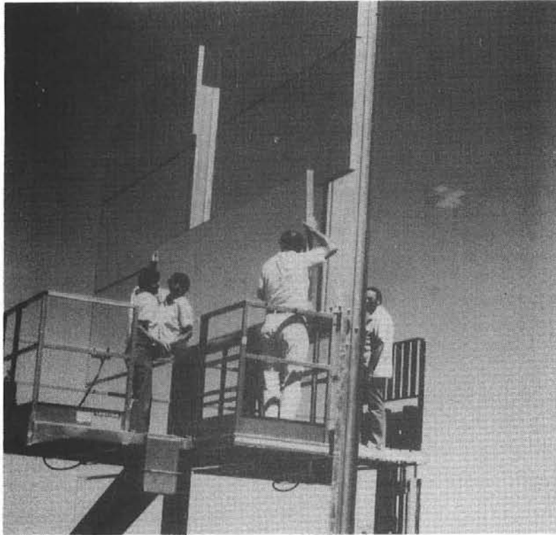
Figure A-3.1. Mirror Modules Being Exchanged on MDAC Heliostat #1
