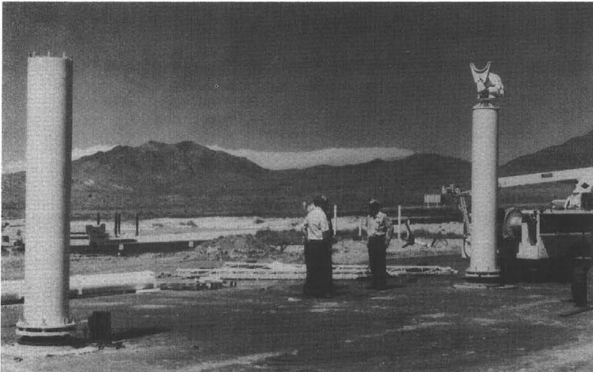
Figure A-15. Field Assembly of MMC Prototype Heliostats
