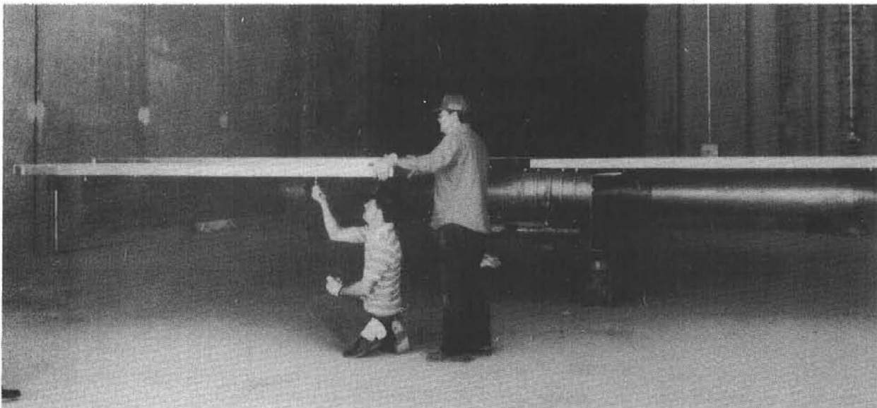
Figure A-2.5. Assembly of MDAC Mirror Modules to the Cross Beams
