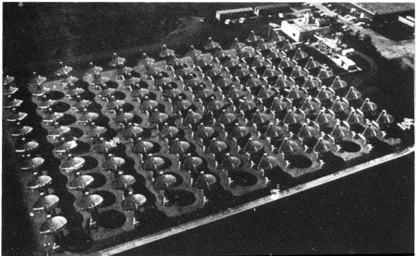
Figure 5. Solar Collector Field, Bleyle Plant Shown in Upper Right
