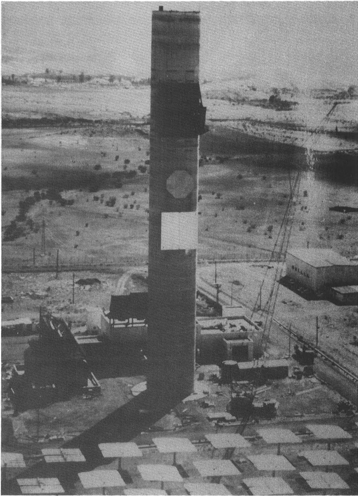
Figure 12. Tower and Equipment Area
