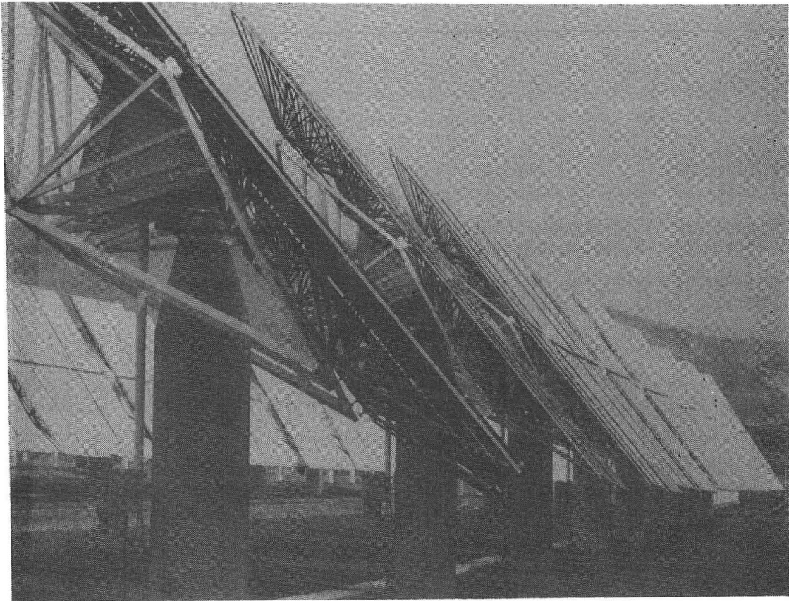
CETHEL Heliostat and Structural Layout
