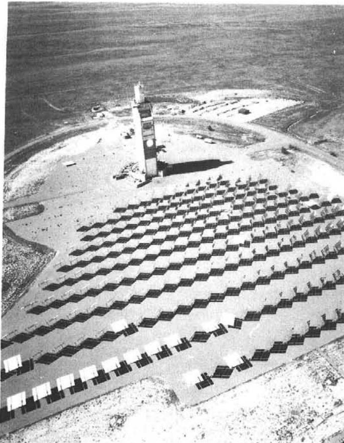
FIGURE 3 AERIAL PHOTOGRAPH OF THE CRTF (with the cavity receiver on the tower)
