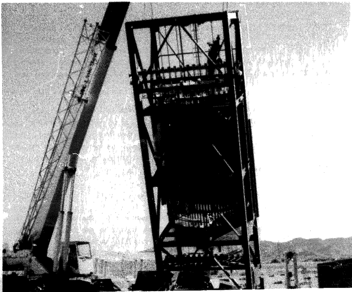
FIGURE 4.2.1 RECEIVER MODULE ERECTION
