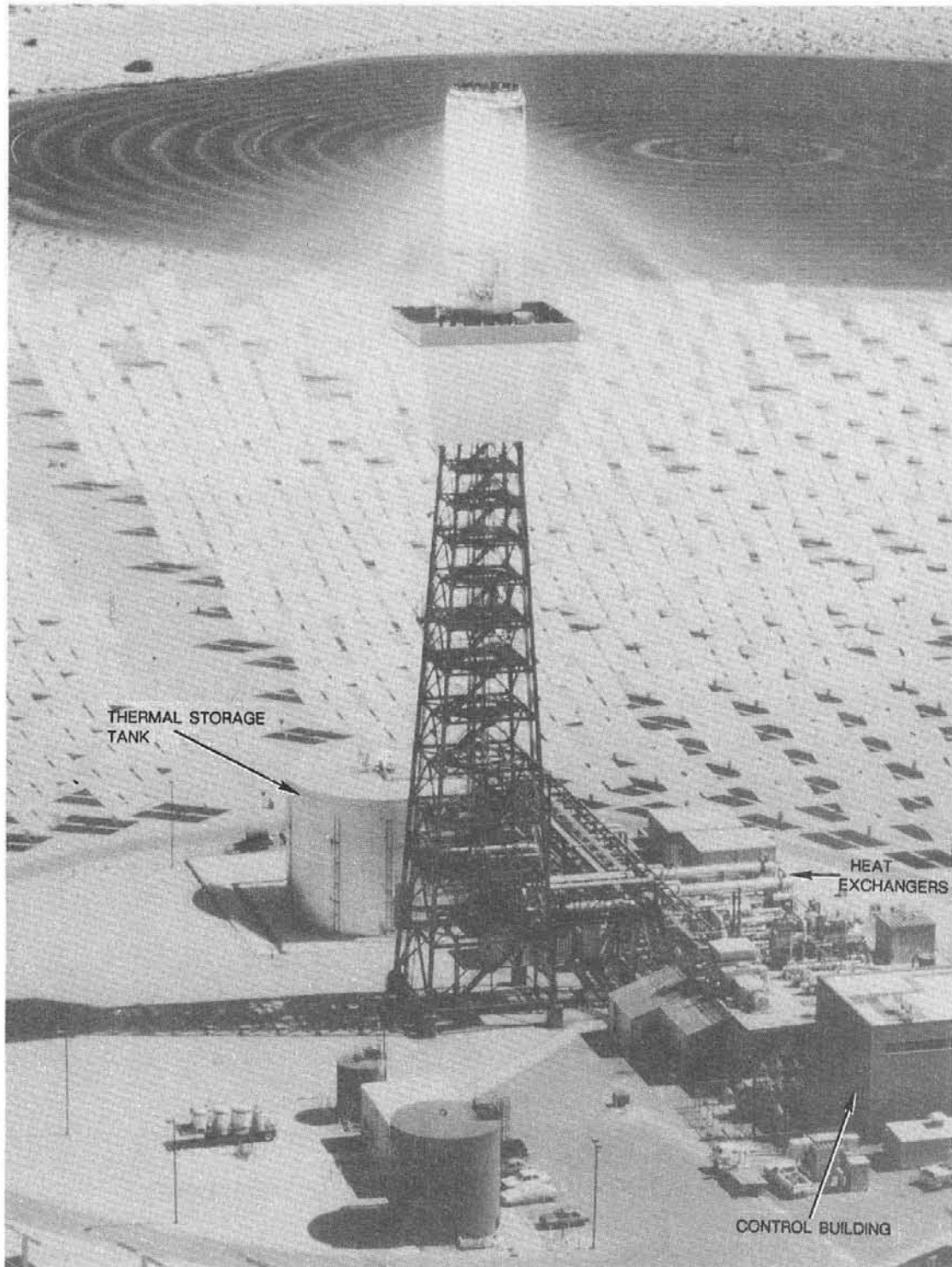
Figure 5. Photograph of the Solar One receiver in operation on the top of a the steel tower. At the base of the tower are the thermal storage tank, heat exchangers, and control building.
