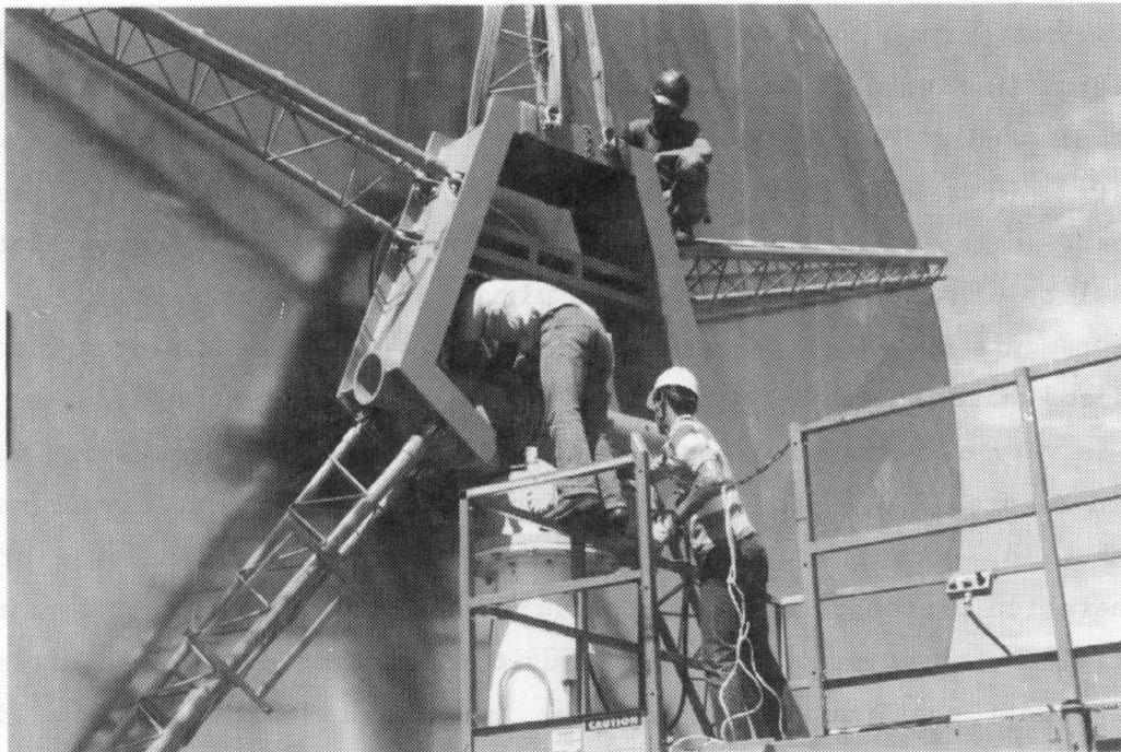
Figure 12.0-22. Installation of Mirror Module (View 3)
