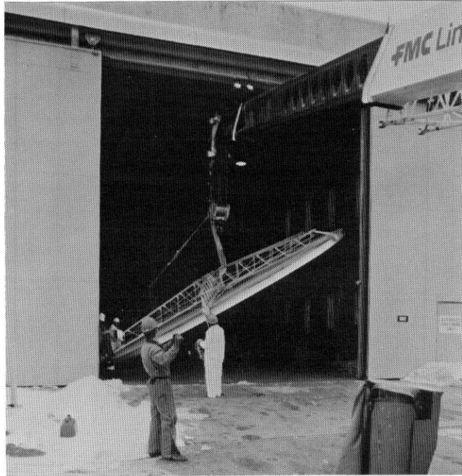
Figure 10.15 Complete Mirror Module Being Rigged Out of Assembly Building at Sandia's CRTF.
