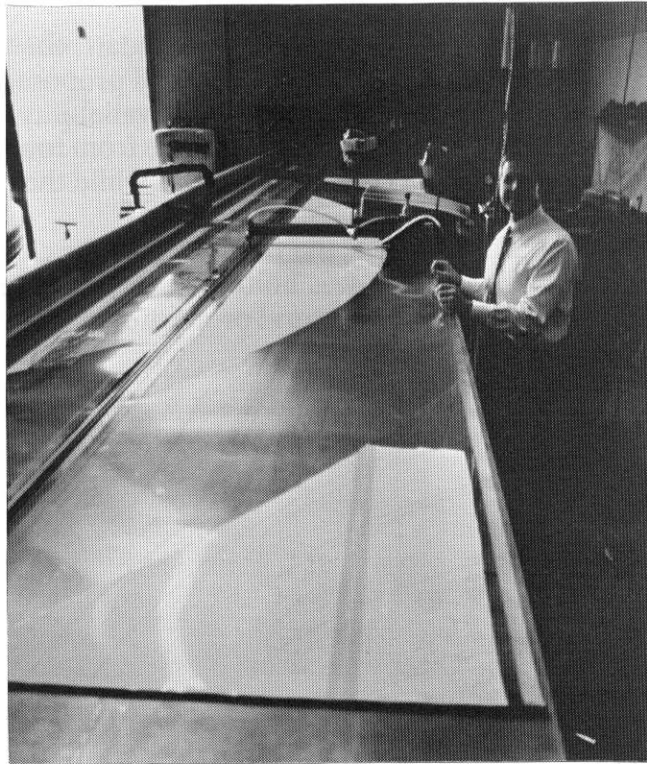
Figure 10.1 Welding Operation for Membrane Fabrication. NOTE: The white circular segment on the membrane panel being fitted is the actual reflective area with a protective premask applied to it. Also visible is the completed 90% of the membrane already rolled up on the shipping mandrel to the left of the welding table. The traveling welder's arms are visible in the background.
