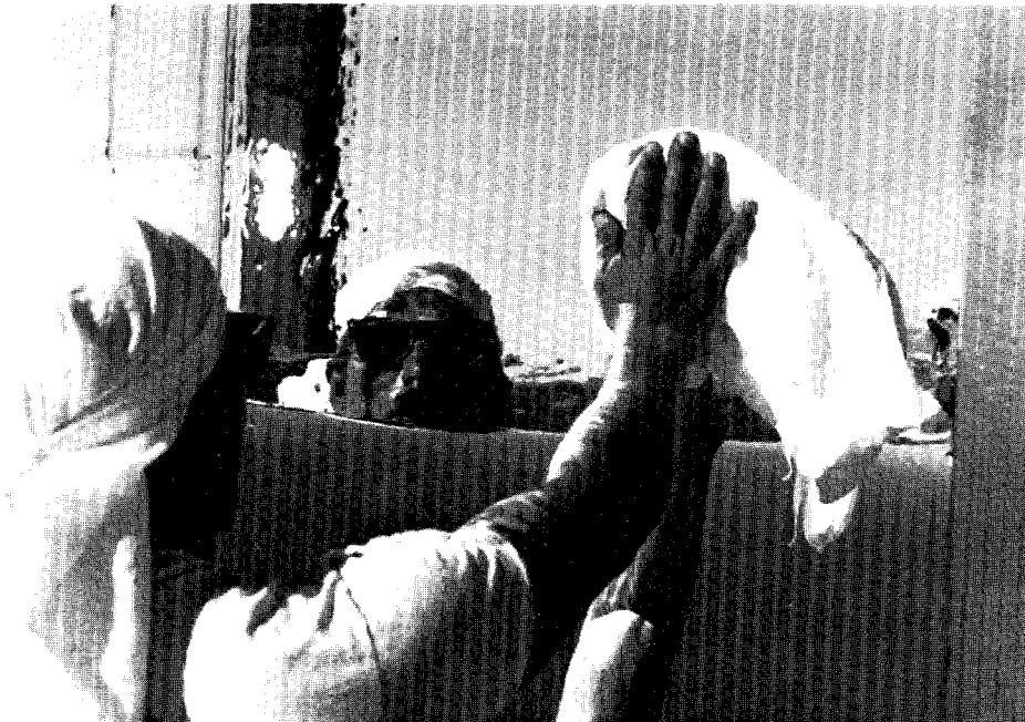
Figure 10 - Smoothing the replaceable reflector into place with a soft cloth
