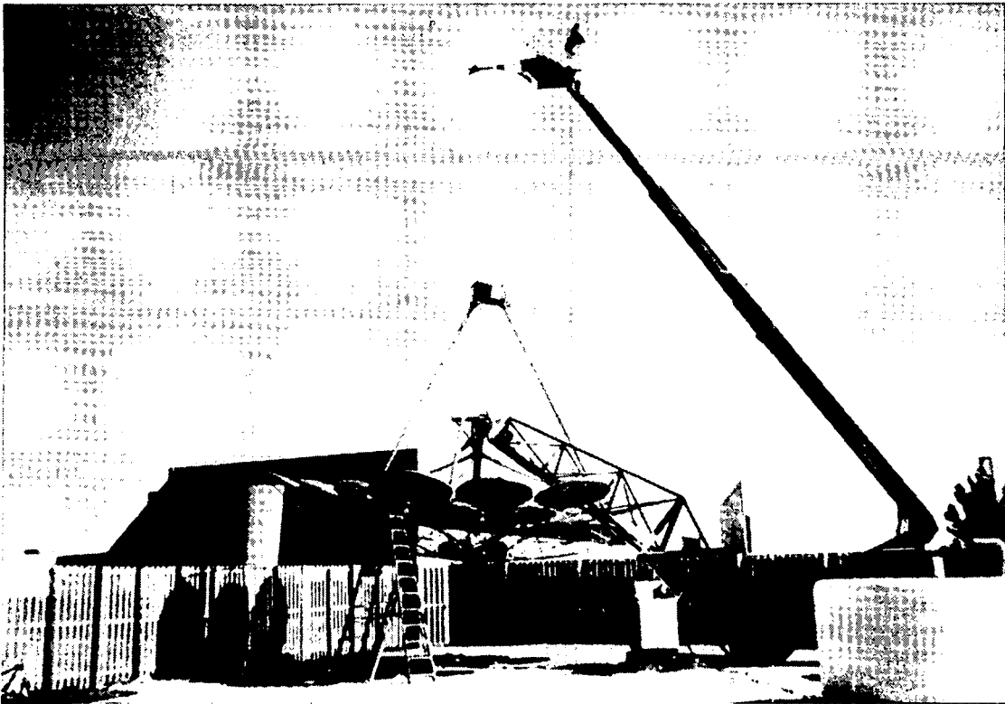
Figure 8. Photograph of the alignment technique adapted to the CPG-460 solar concentrator.
