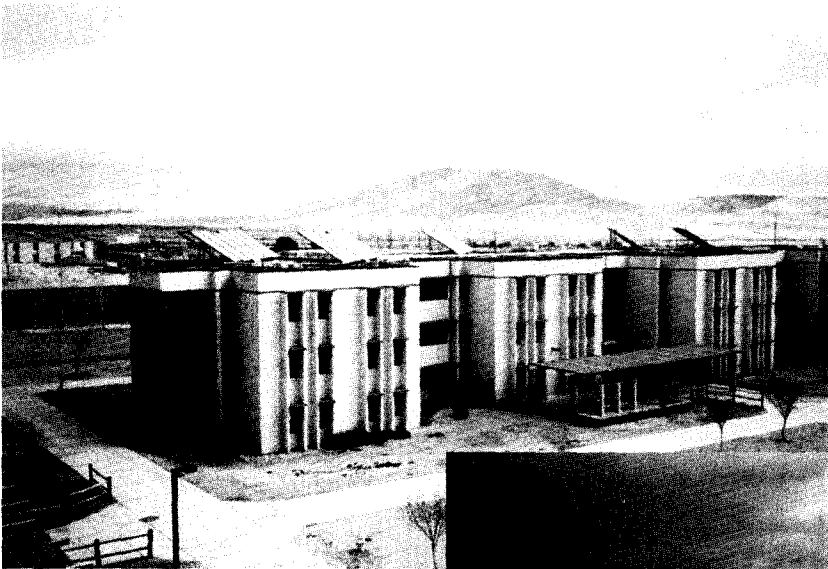
Solar system at the Bachelor quarters at Fort Irwin Army Base, California.
