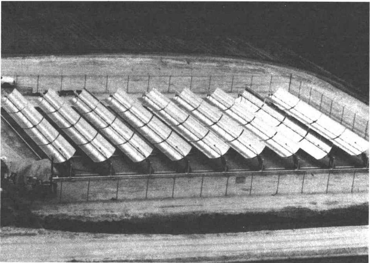
FIGURE 2. THE NML/BMI 50-HORSEPOWER SOLAR-POWERED IRRIGATION SYSTEM: 1977
