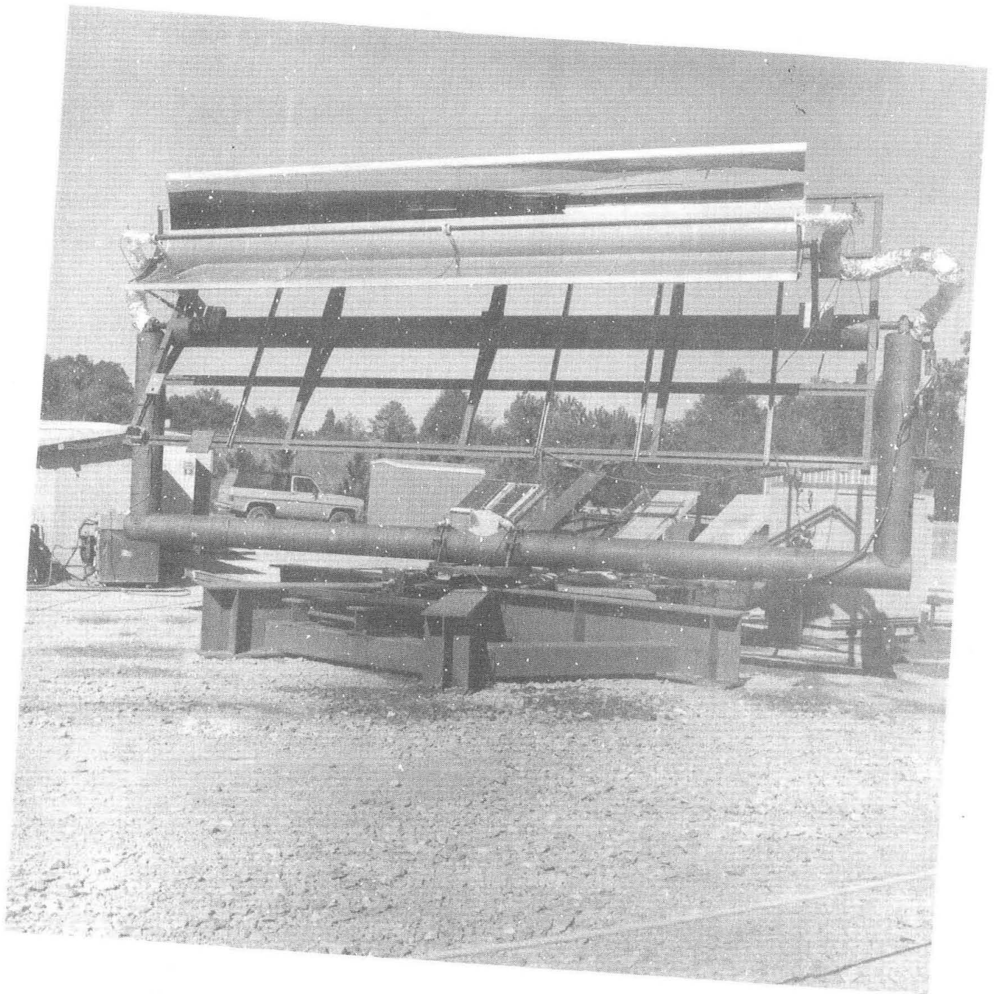
Figure 1. Solar Kinetics T-600 Solar Collector
