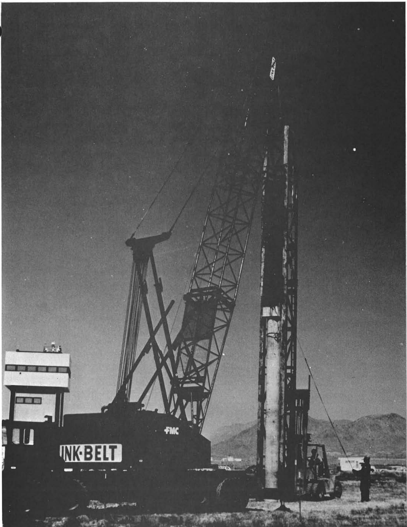
Figure 4.3-1. Pile-Driver and Pedestal - Site B2
