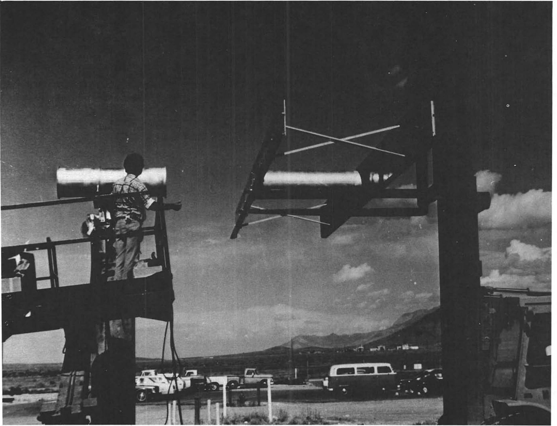
Figure 4.3-6. Installation of an H-Frame Assembly
