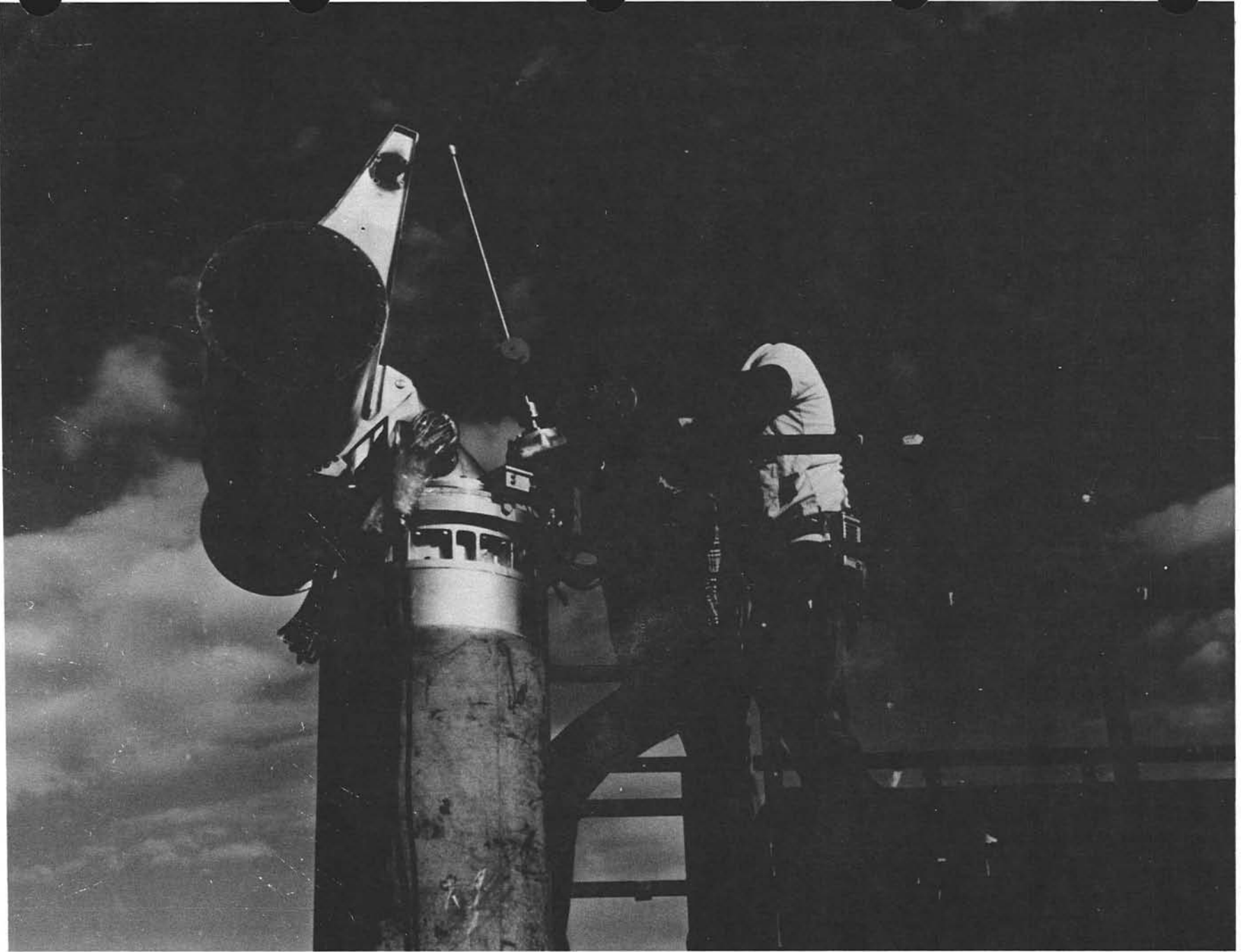
Figure 4.3-5. Installation of Elevation Drive
