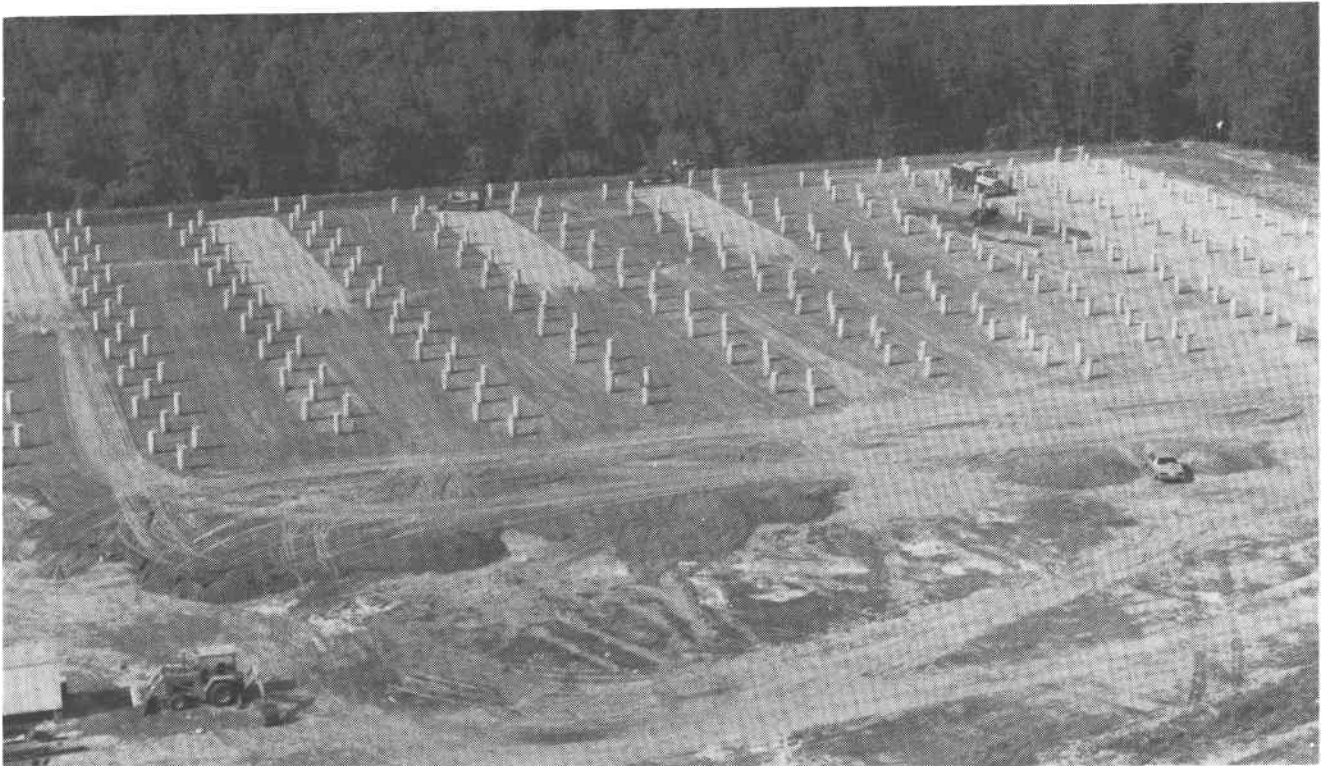
Figure 6. Collector Field Under Construction, April 1981
