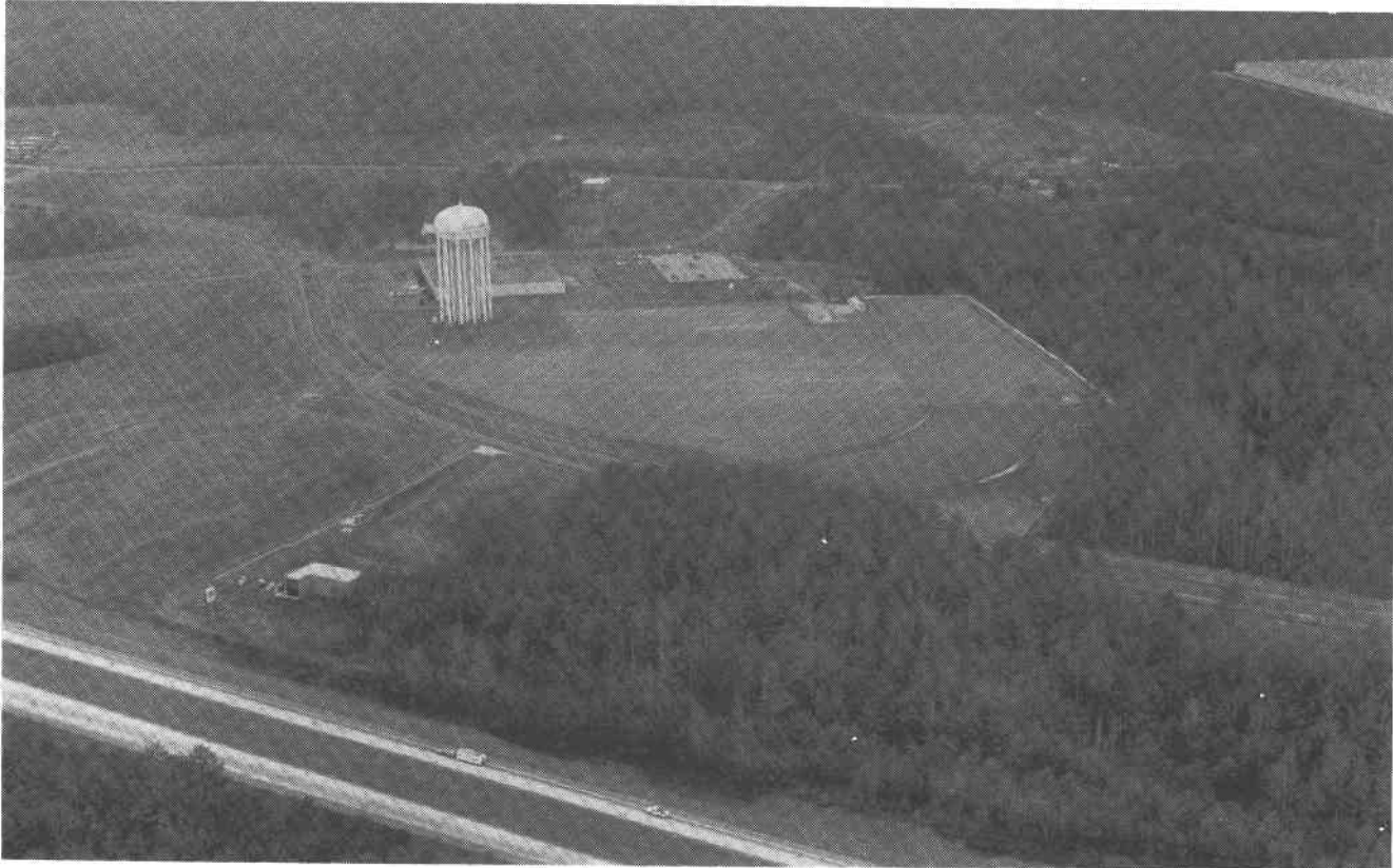
Figure 4. Site Initial Preparation, March 1980
