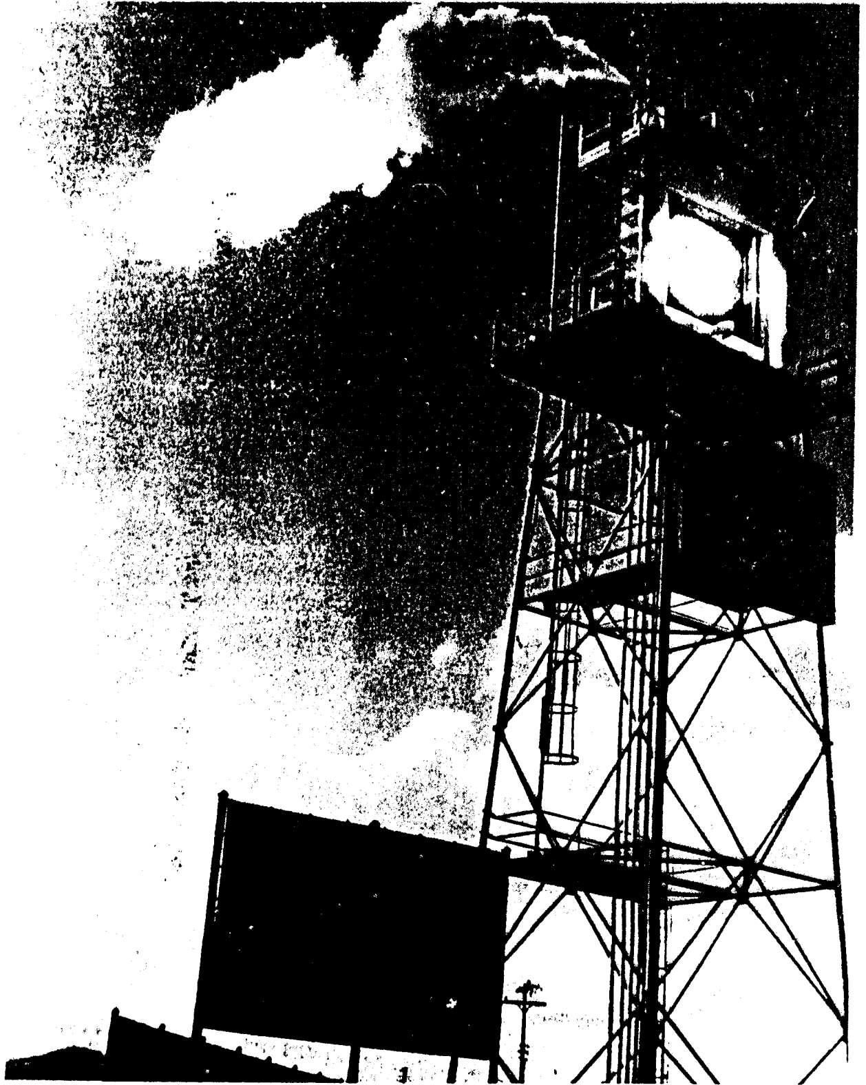
FIGURE I-6 RECEIVER OPERATING DURING SYSTEM STARTUP
