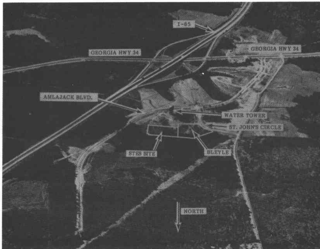
Figure F-3. Aerial Photograph - Looking South
