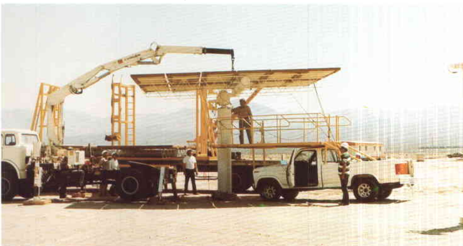
Mounting of Heliostat on Pedestal
