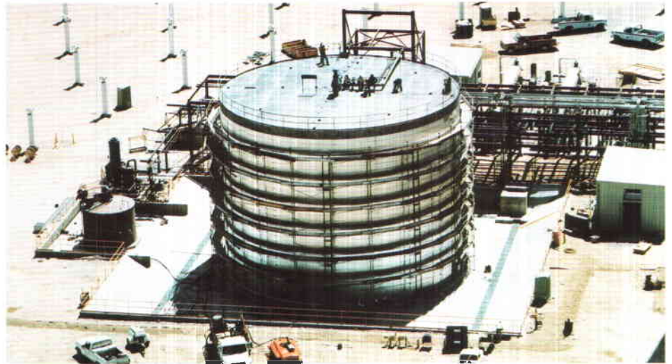
Construction of Solar One's Thermal Storage System
