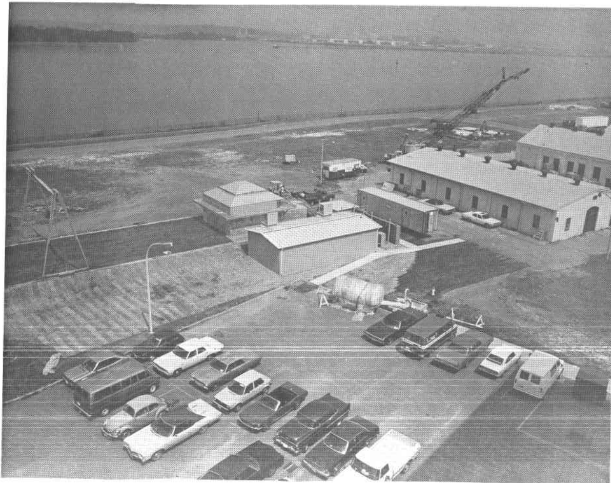
Fig. 21 — Aerial view of energy storage boiler tank at the Naval Research Laboratory. The storage tank is located inside the square structure closest to the river. An adjacent Butler building provides storage for Dacotherm insulation, which can be removed from around the hot tank to facilitate repairs or alterations. An instrument trailer is located next to the facility to process data and to relay information to a nearby laboratory building. The storage facility is serviced by a lightweight gantry crane. The layout permits construction of a second experimental tank at the same site.
