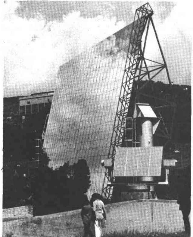
(a) 13.5x17.0 m (44.3x55.8-ft) HELIOSTATS AT CNRS FACILITY SHOWING MASSIVE STRUCTURAL REQUIREMENTS
