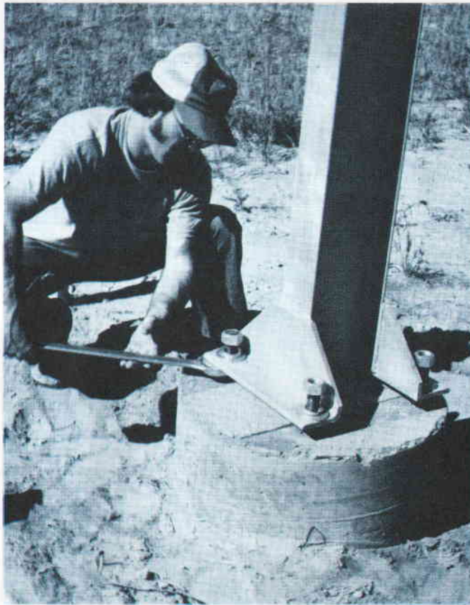
Figure33. Double-Nut Technique Used for Adjustment of Support Pylons
