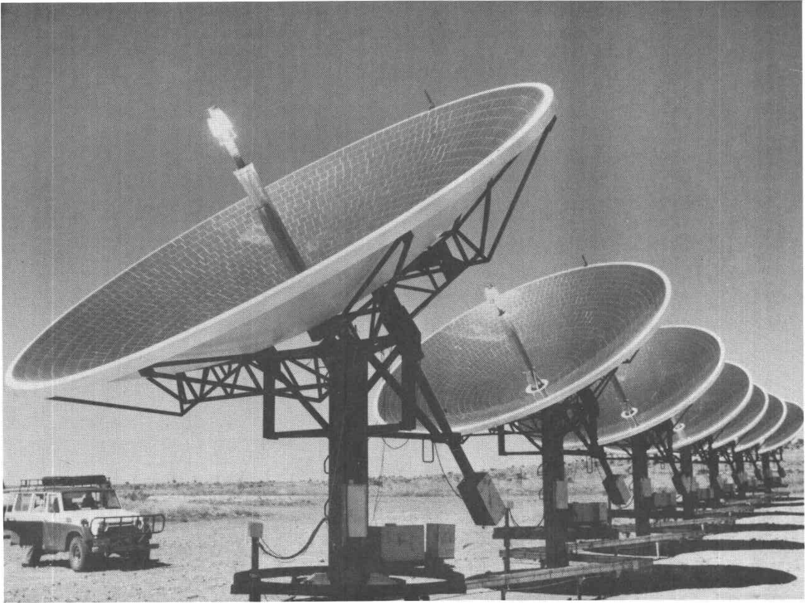
Figure 1(a). Paraboloidal Dishes at White Cliffs Solar Power Station, Australia
