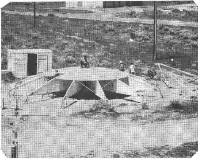
FIGURE 5. PARTIAL DISH ASSEMBLY
