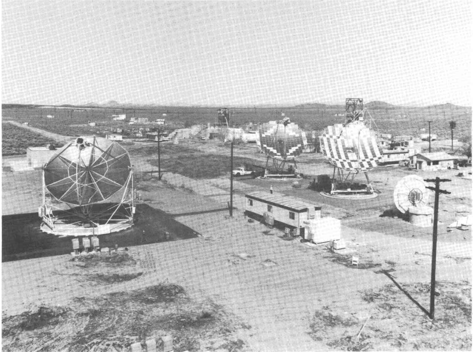
Figure 12. Parabolic Dish Test Site. (PDC-1 is on the left; the two TBCs are on the right.)
