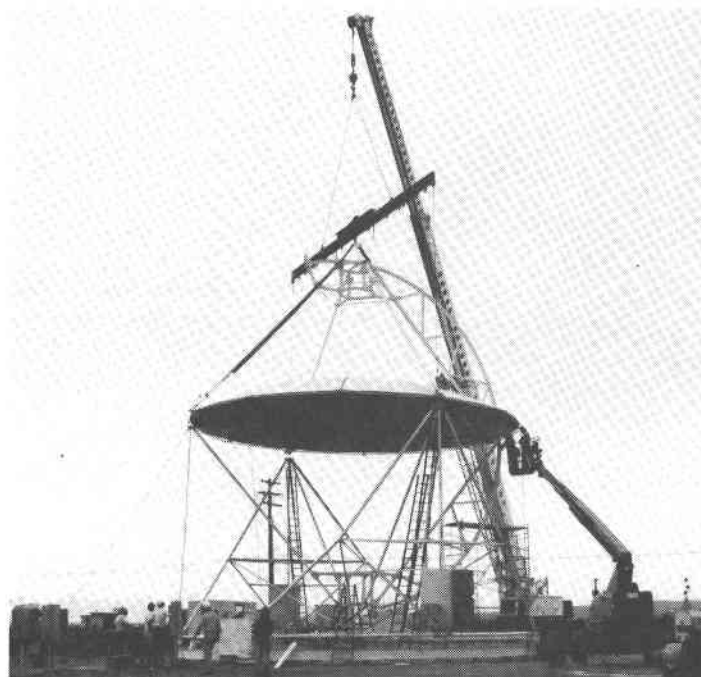
Figure 3-4. Dish Assembly Positioned Over Base Frame by Crane
