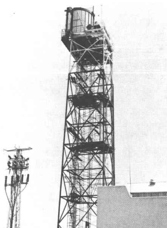
Central Receiver Tower at Small Solar Power System Project in Almeria, Spain
