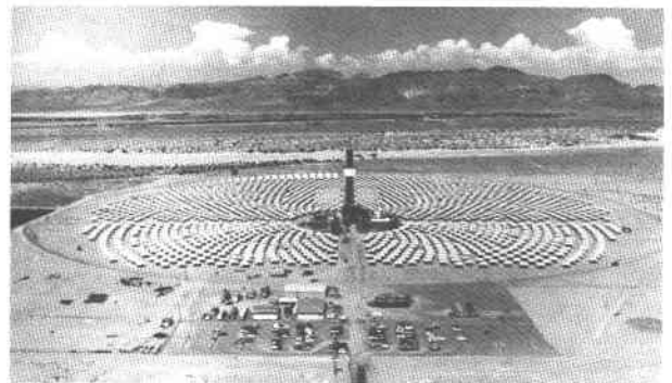
Heliostat Field at 10-MWe Solar Central Receiver Pilot Plant Near Barstow, California
