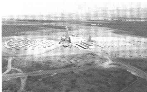
Field of Heliostats and Parabolic Troughs at Small Solar Power System Project in Almeria, Spain
