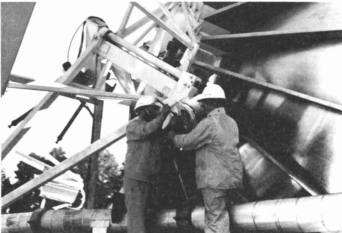
Figure 3-5. Replacement of Corroded New Stainless Steel Tubing
