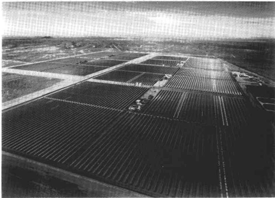
Figure 9. Aerial view of the five SEGS plants located at the Kramer Junction Power Park. The plants produce 150 MW of electricity and comprise 1 million square meters of glass.
