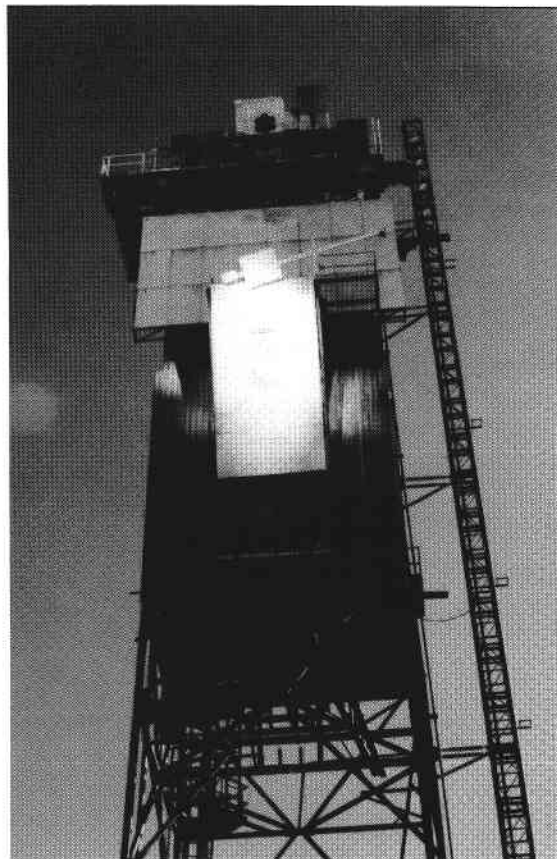
Figure 14. Internal film receiver being tested at Plataforma Solar de Almeria, Spain.
