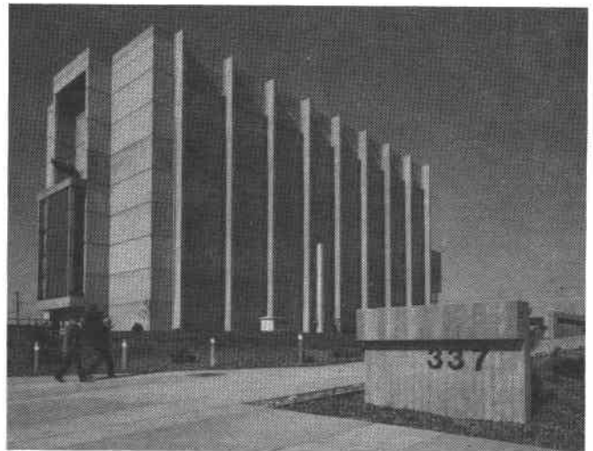
Figure 1. Exterior View of HTSF building
