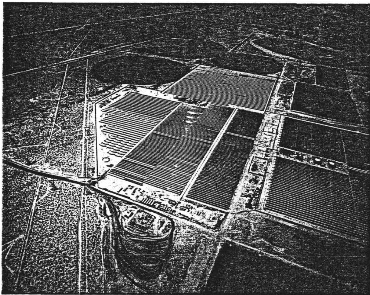
Figure 20. The Solar Electric Generating Station (SEGS) at Daggett, California
