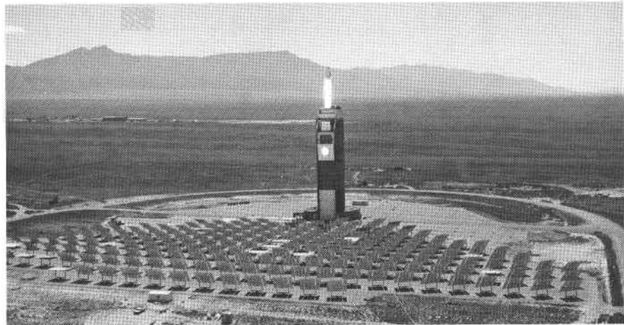
Central Receiver Test Facility in Albuquerque, New Mexico.
