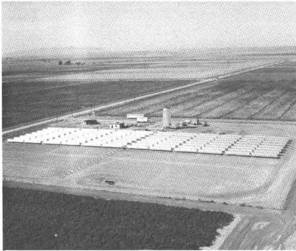
Figure 3-13. Deep-Well Irrigation, Coolidge, Ariz.
