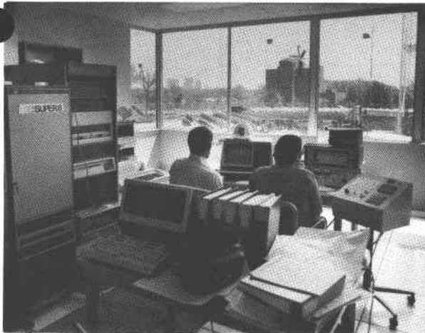
Figure 4-13. Advanced Components Test Facility Control Room
