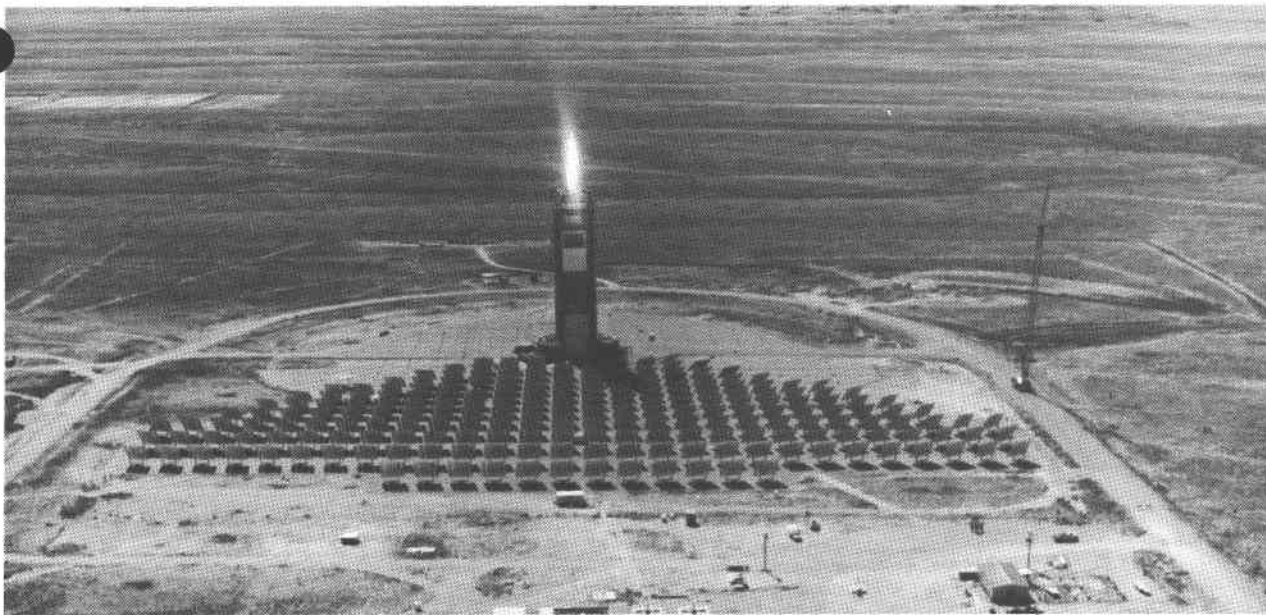
Figure 2-12. Central Receiver Test Facility
