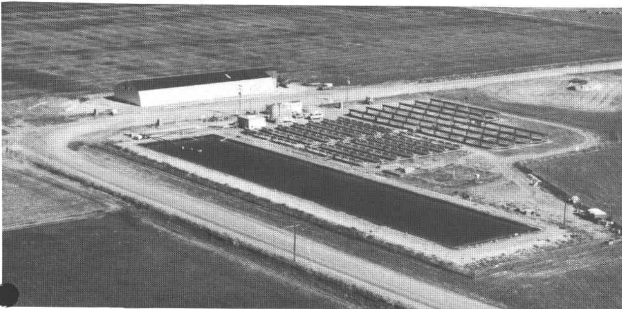
Figure 3-12. Shallow Well Irrigation, Willard, N.M.
