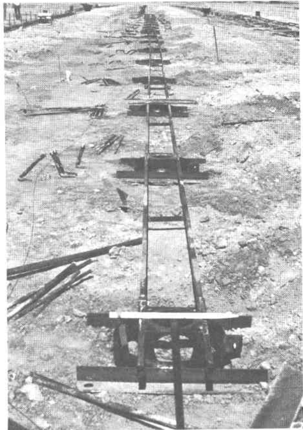
Figure 94. Collector Foundation Template, Coolidge Facility
