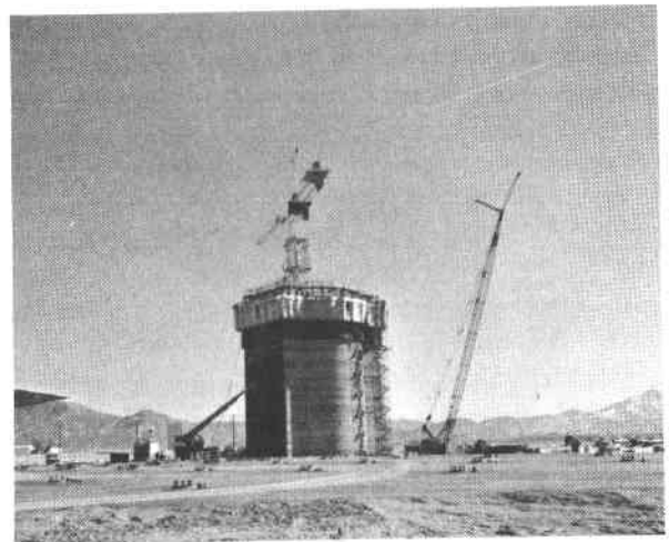
Figure 134. CRTF Tower Construction
