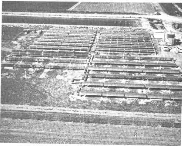
Figure 88. Willard Solar Irrigation Facility with the Installation of Additional Collectors and Thermal Storage Nearing Completion
