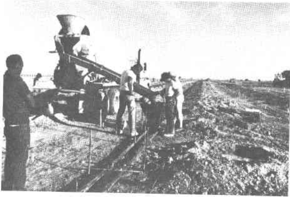
Figure 95. Pouring Collector Foundations at Coolidge
