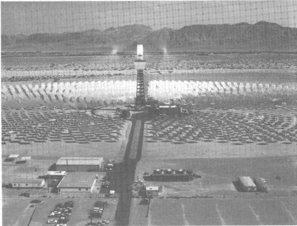
Figure 1. The 10-MWe Central Receiver Pilot Plant near Barstow, California
