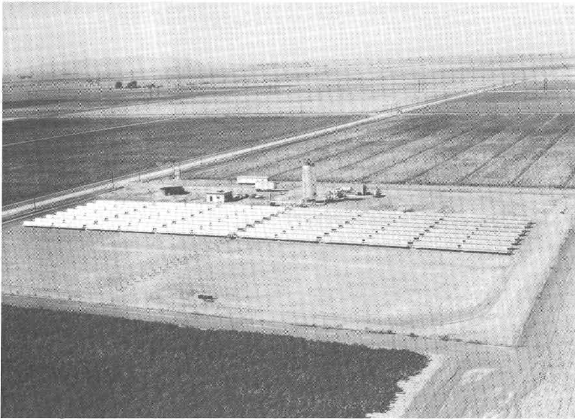
Figure 11. 150-kWe Solar Irrigation Project, Coolidge, Arizona
