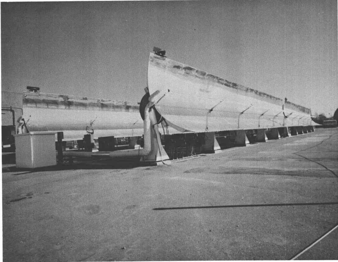
Figure 5-4. Line-Focus Distributed Receiver Concept Using Parabolic Troughs
