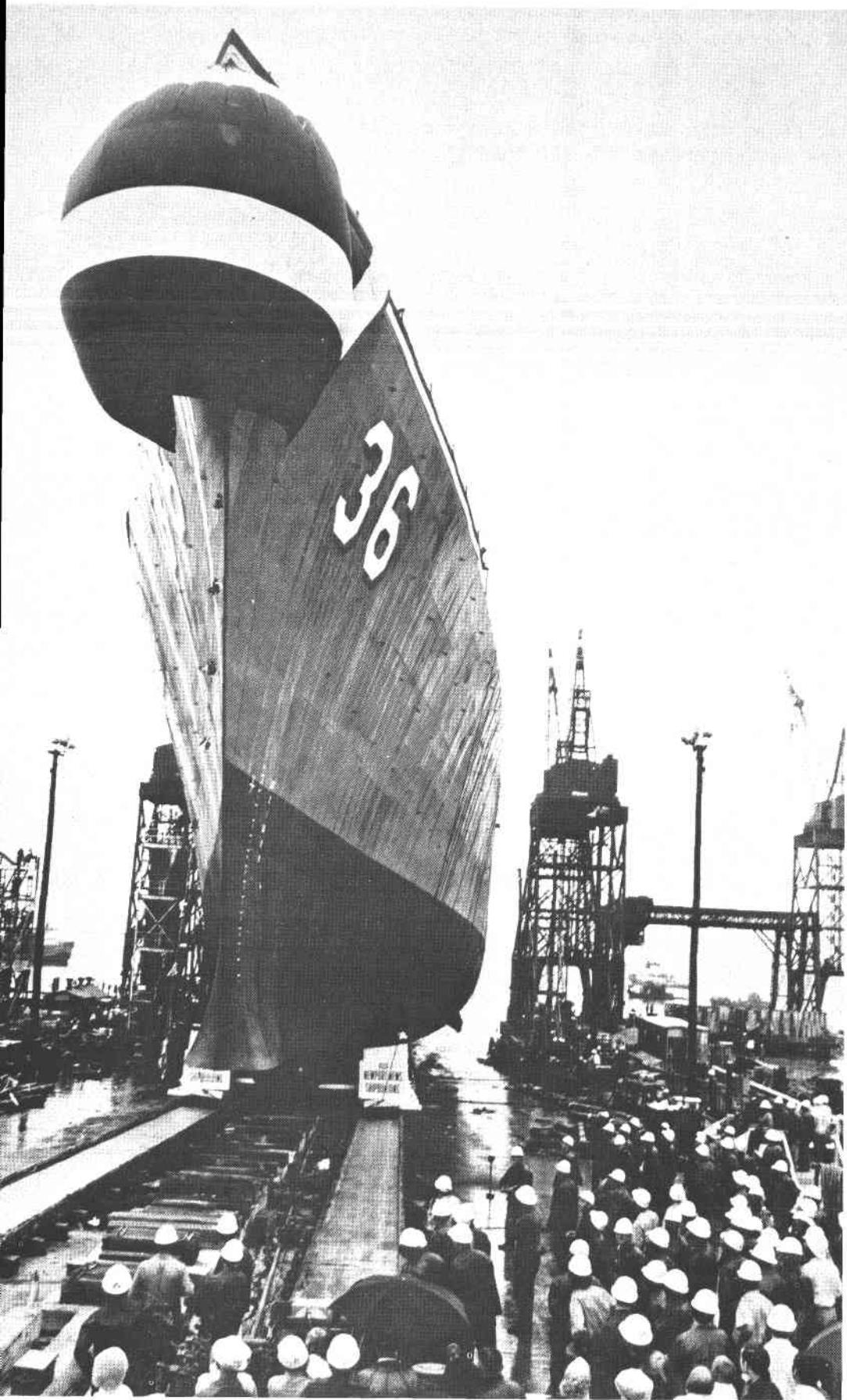
The nuclear powered guided missile Frigate California (DLGN36) is shown as it slides down the ways during the launching ceremony at the Newport News, Va.
