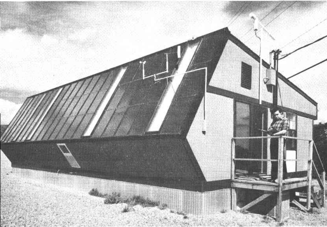
Exterior view of the laboratory under construction.
