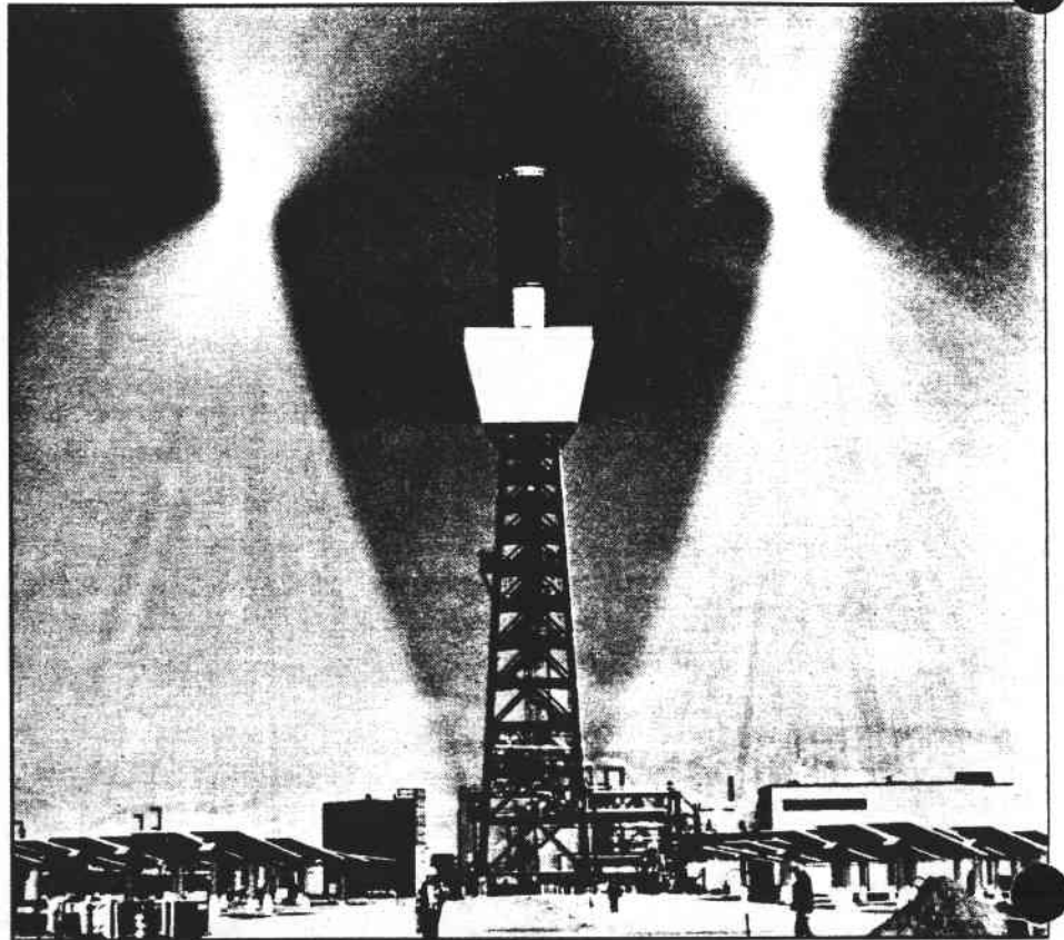
A spectacular display of light is evident when dust or moisture in the air is lit by hundreds of heliostats at Solar One. The world's largest solar-powered electrical generating station began "startup" tests early this spring and recently generated its first electric power. Each morning, heliostats reflecting the sun's rays are first focused on "stand-by" points, and then moved onto the receiver to create steam to operate the turbine-generator below.
