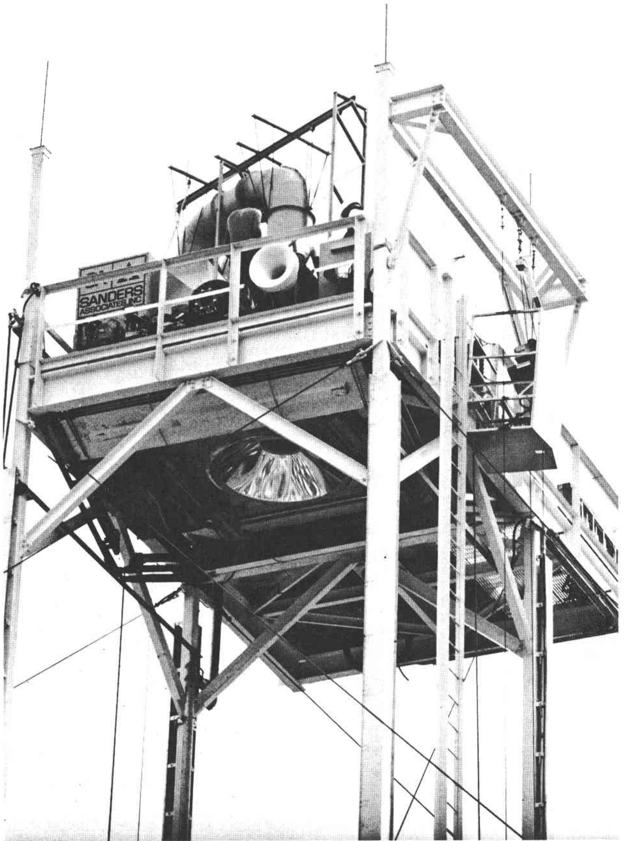
Figure 2-2. Receiver and Concentrator 2-4
