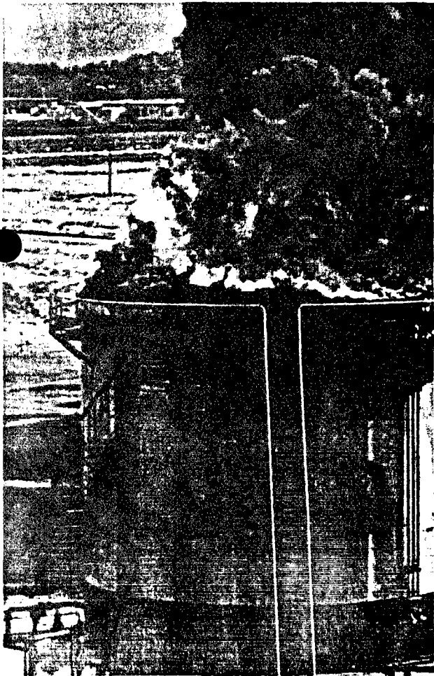
Typical storage tank fires can cause massive property and personal loss
