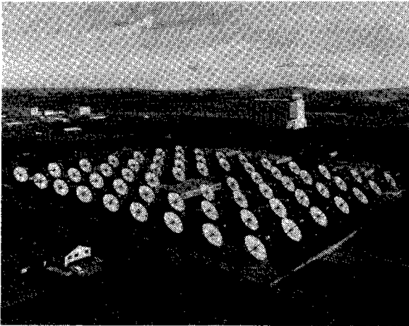
FIG. 5 EXAMPLE OF A 1-MWe SMALL COMMUNITY SOLAR THERMAL POWER EXPERIMENT
