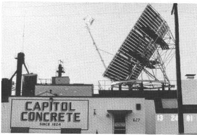
Figure 1.7. Power Kinetics, Inc., point-focus concentrator producing process heat at Capitol Concrete Co. in Topeka, Kans.
