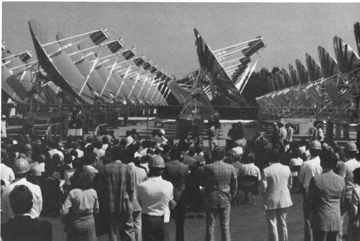
STEP in Operation at Shenandoah, Georgia
