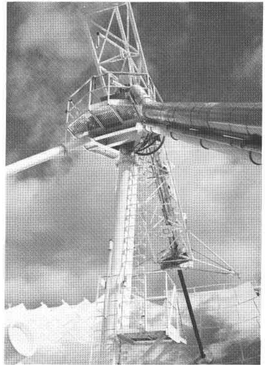
Receiver Assembly of Hemispherical Bowl near Crosbyton, Texas. The water inlet and steam output lines are visible in the foreground.
