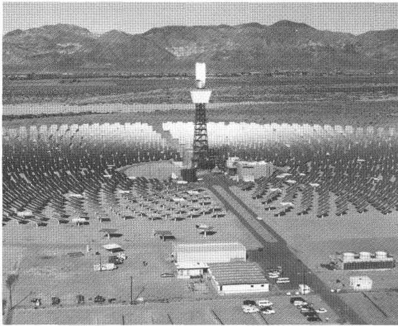
Solar One in Operation
