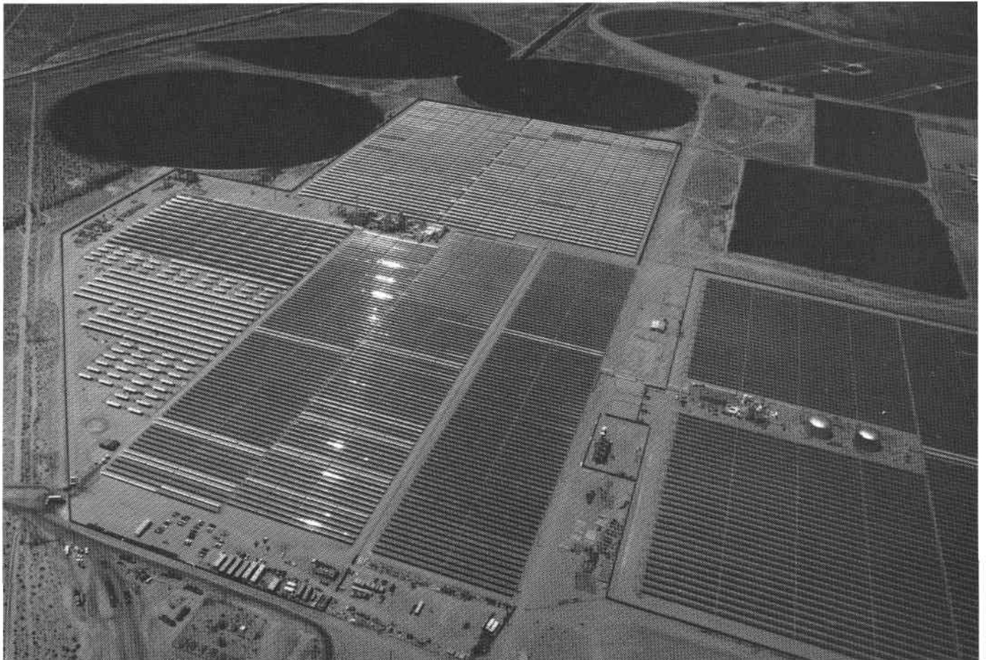
Figure 2.5. The Solar Electric Generating Station (SEGS) at Daggett, California
